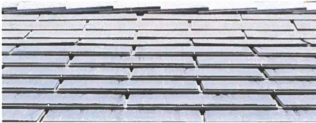
Solar shingles attached to the front exterior of the shingle. Photo courtesy City of Santa Barbara
