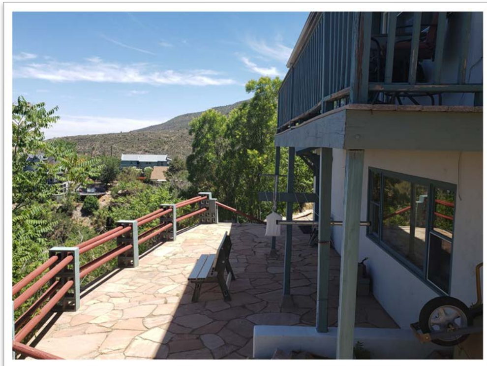
Existing deck and patio - note that patio extends across rear property line.
