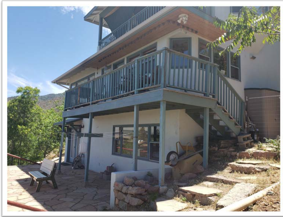
Existing deck that extends 5' from house
